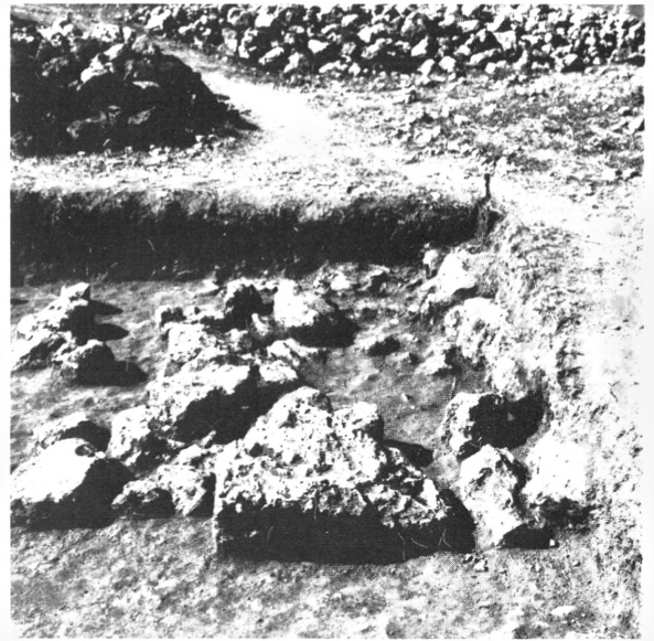
Fig. 8. F 11 NW. The “northern wall” as seen from the east.
