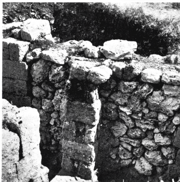
Fig. 140. Complex XII. Door between rooms 35 and 36 as seen from the south-east.
