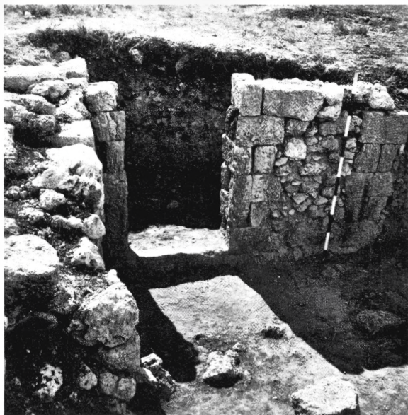
Fig. 139. Complex XII. Room 35 as seen from the north-west.
